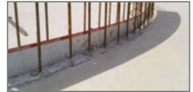
with curing compound
