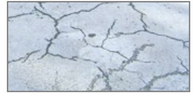
without curing compound
