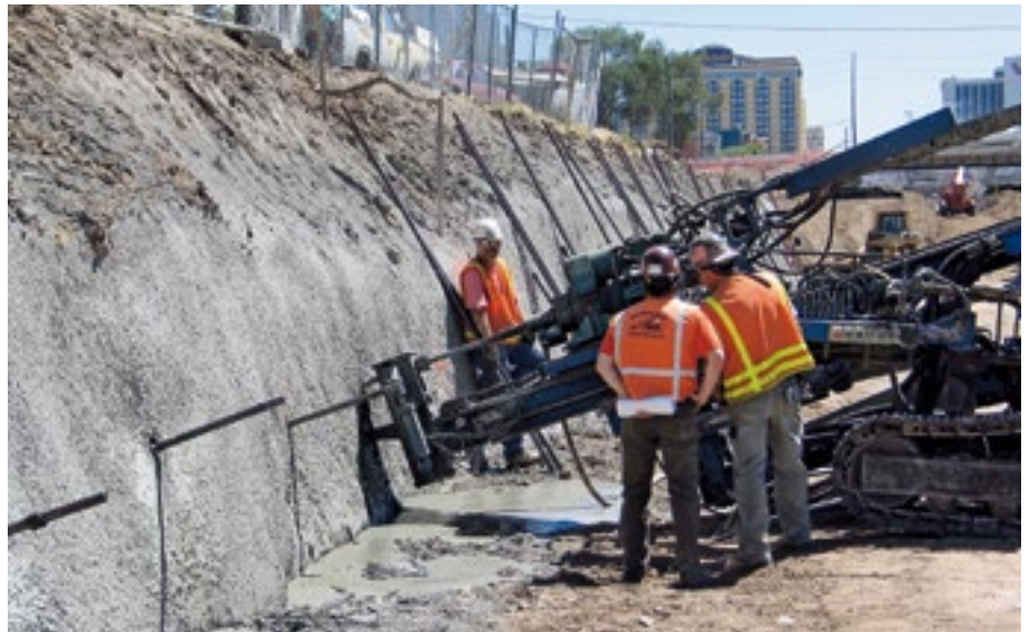
Stabilization of a trough structure using DYWI® Drill Hollow Bar Anchors, Ø 38mm – Reno, Nevada, USA
