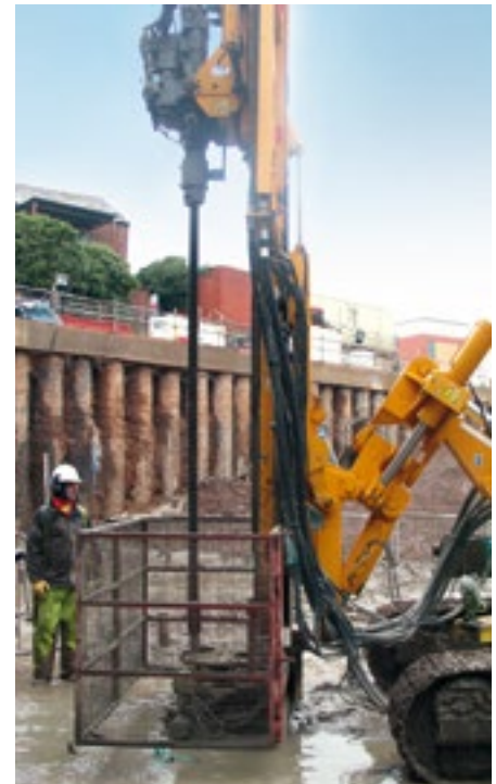
Long stroke drill boom for deep micropiles
