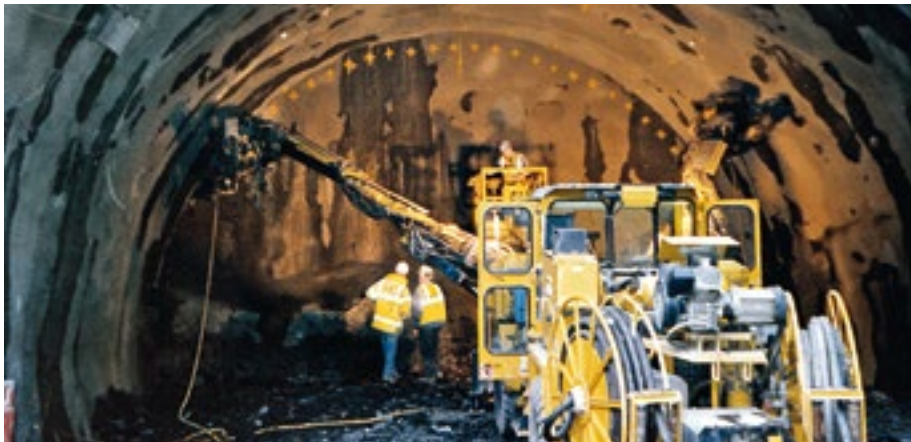
DYWI® Drill hollow bar spiles for the stabilization of a launch adit for a TBM
