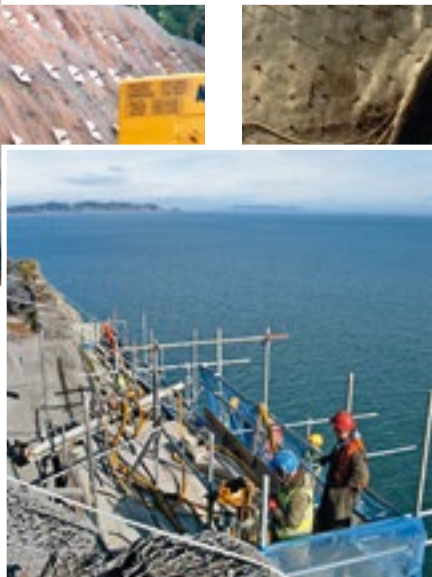
Scaffold mounted hydraulic drill boom for rock bolting
