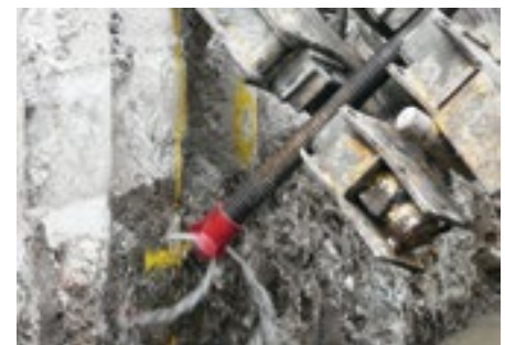
T76 ESS-D 130 drill bit for rock sockets, also for drilling through (soft) secant piles
