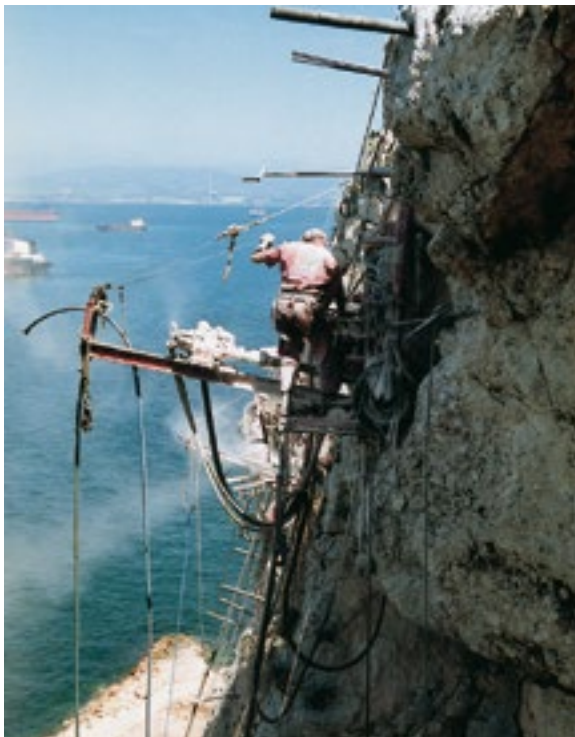
Slope stabilization using DYWI® Drill Hollow Bar Anchors at the Rock of Gibraltar
