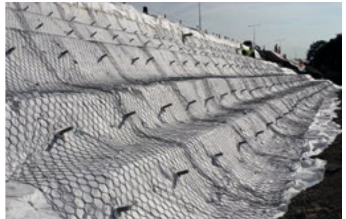
Benched face stabilised with DYWI® Drill soil nails
