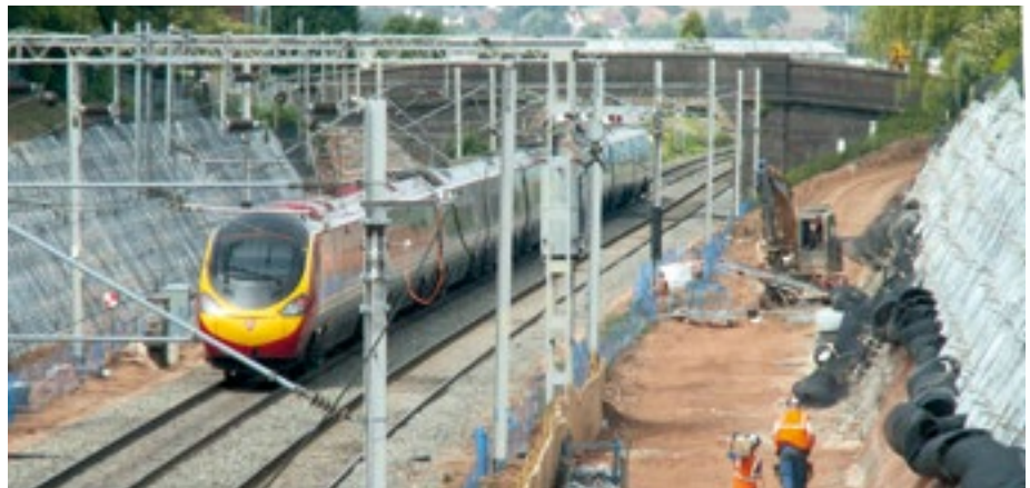
DYWI® Drill Galvanized hollow bar soil nails for railway cutting widening
