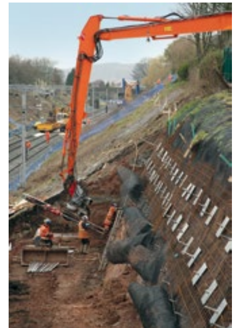
Long reach excavator for restricted access drilling
