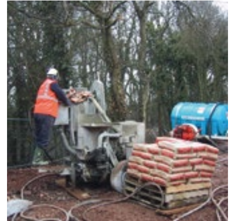
Grout pump with colloidal mixing unit
