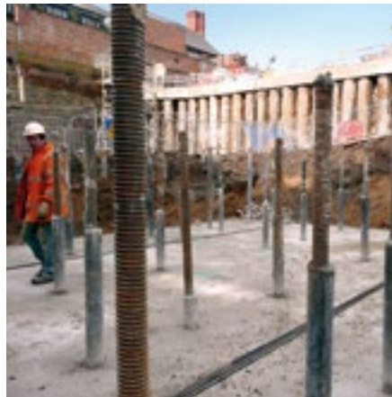
DYWI® Drill T76 micropiles with in-situ steel tube over top 2m
