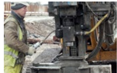
Greasing of seal tracks (H64/R51 adaptor)
