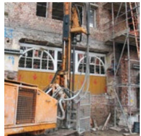
Micropiles for retained facade frame bases
