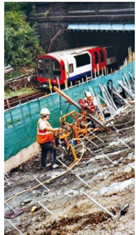
Restricted access soil nailing
