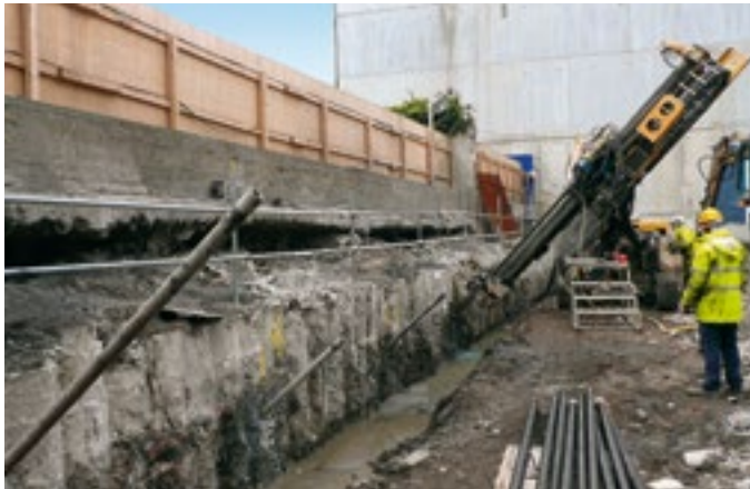
Drilling through a secant piled wall
