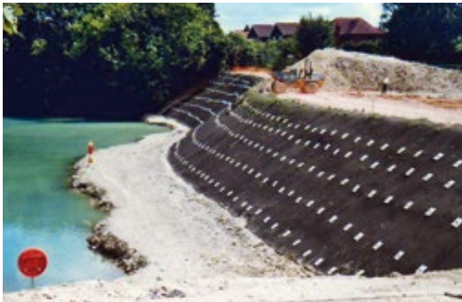
Flexible reinforced geogrid, with vulcano bearing plates for angle compensation
