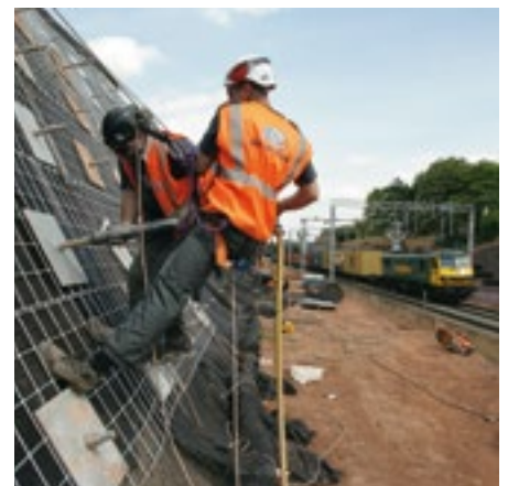
Plating up, using pneumatic box wrench
