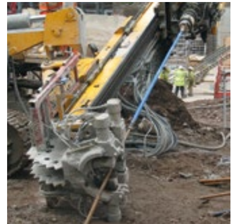
DYWI® Drill free length system for temporary anchors
