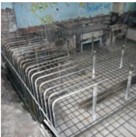
Base slab reinforcement using micropiles
