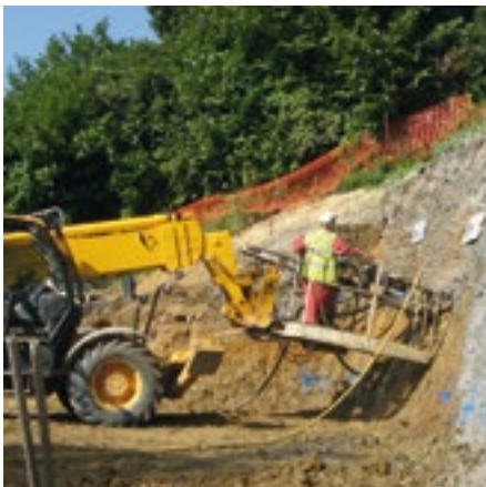
Drill platform mounted on telescopic forklift
