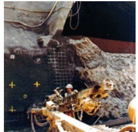
Drilling of hollow bar rock bolts in variable ground
