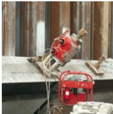
1,500kN jack for T76 temporary anchors
