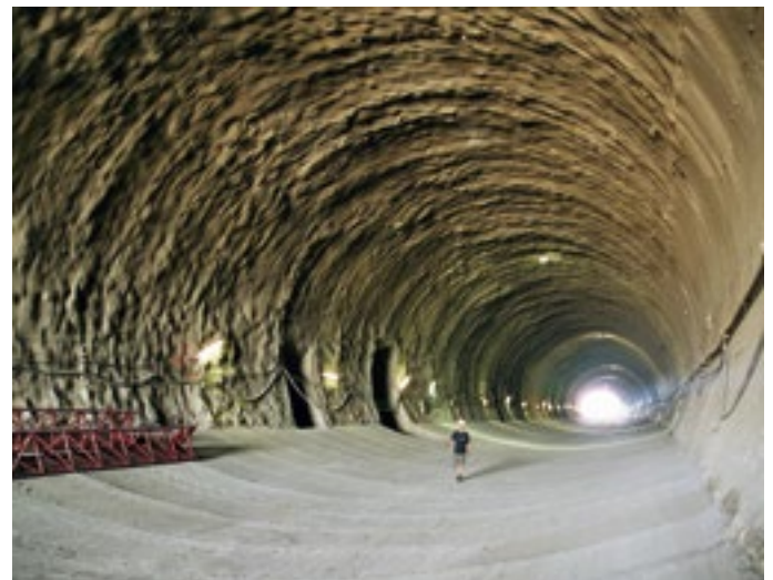
Installation of 67,000m of DYWI® Drill Hollow Bar Anchors, Ø 25mm – Valik Tunnel near Pilsen, Czech Republic
