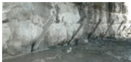
Raking micropiles for bridge pier upgrades
