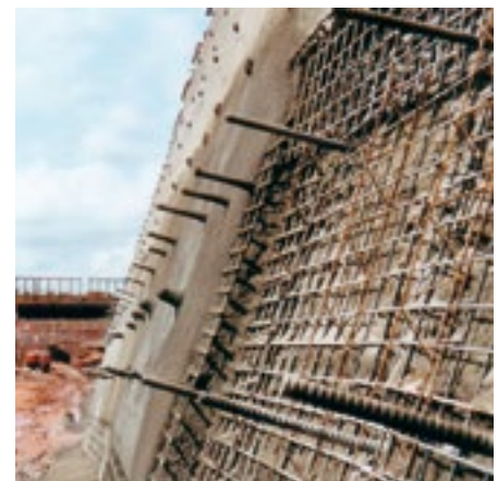
Grouted soil nails on shotcrete face
