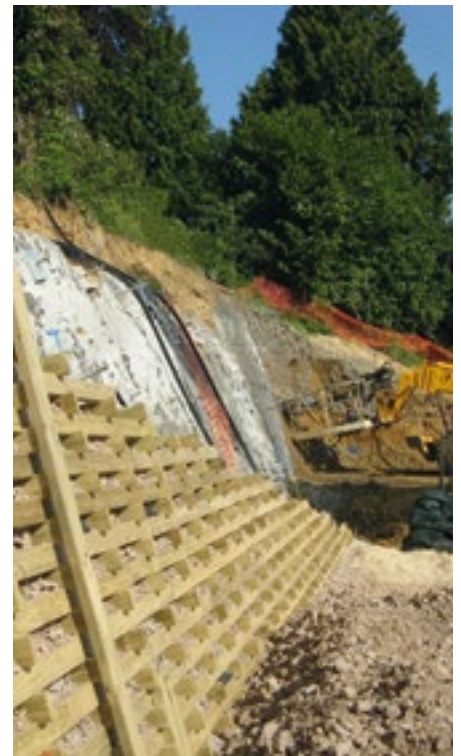
Soil nailed slope with crib wall facing
