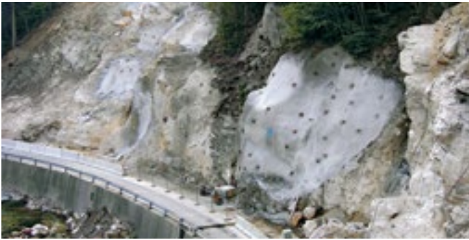
Slope stabilization following a rock fall – Carinthia, Austria
