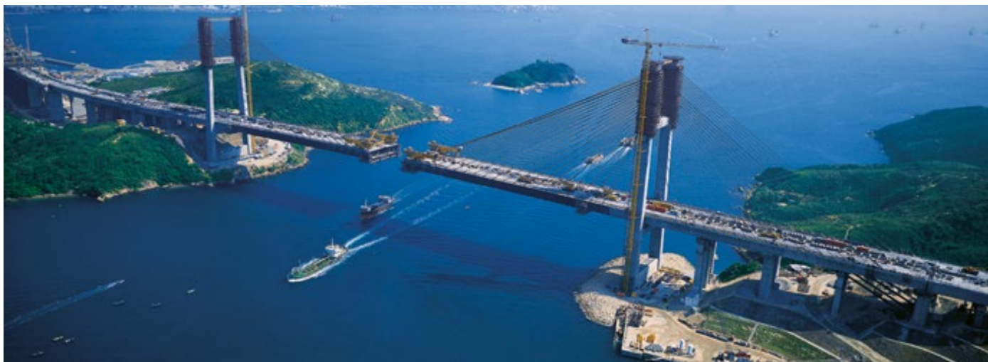
1995: Kap Shui Mun Bridge, Hongkong, China DYNA Bond® Stay Cable Bridge with 176 cables
