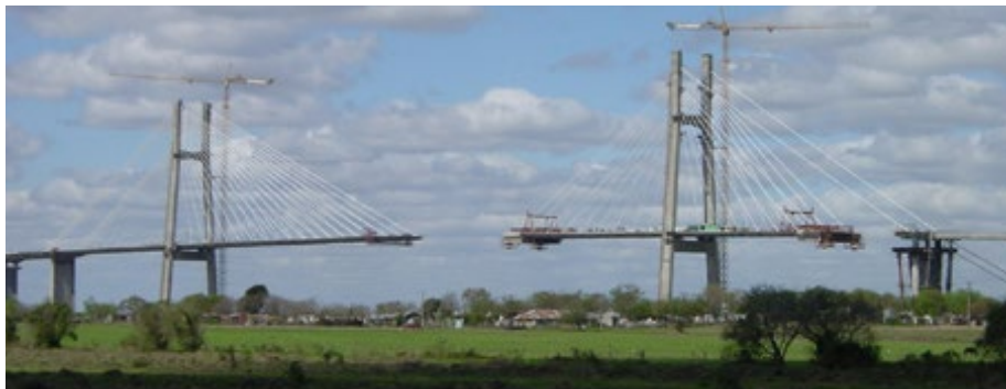
2000: Victoria Bridge, Rosario, Argentina First DYNA Grip® Stay Cable Bridge
