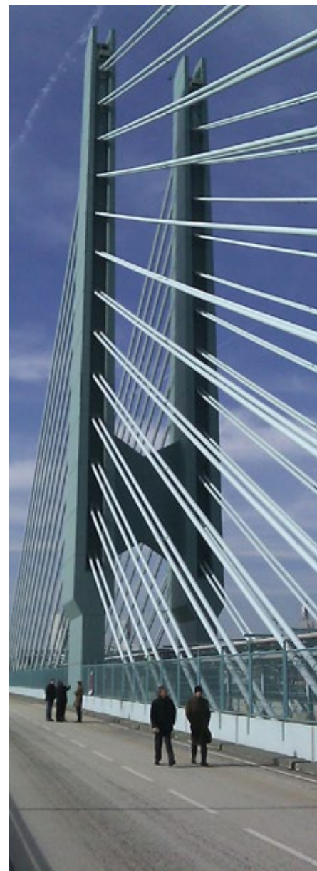
1972: 2. Main Bridge, Hoechst Chemicals, Frankfurt, Germany
