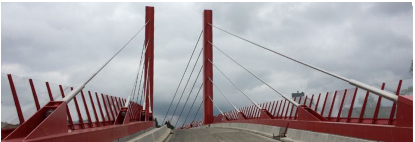
Stainless Steel Duct
