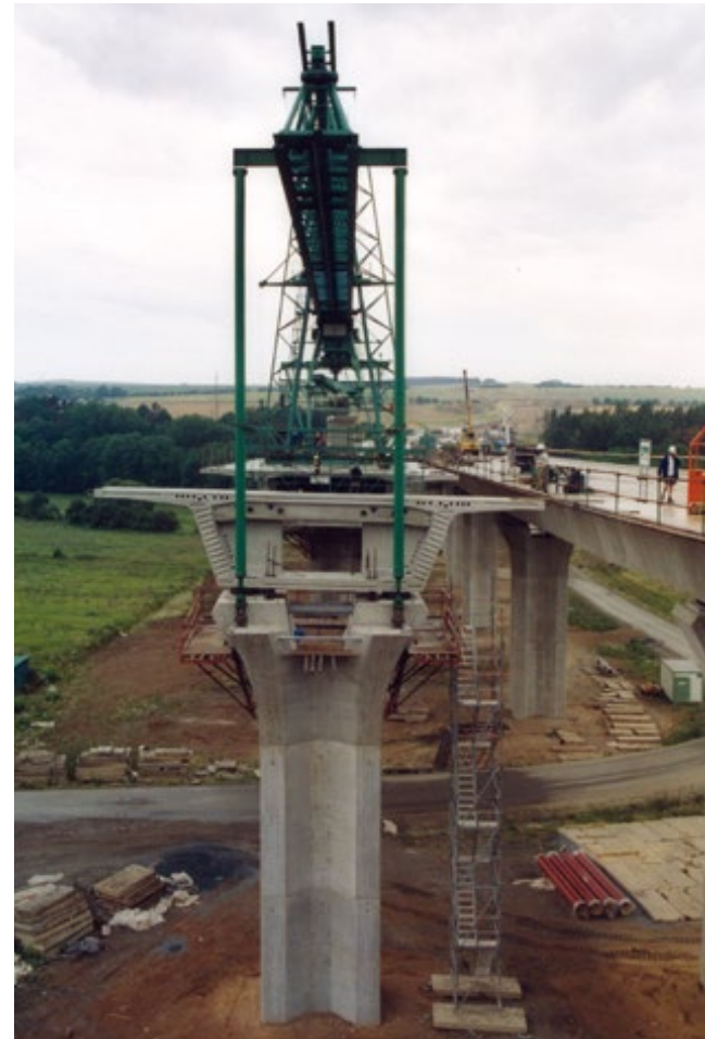
Uhlavu Bridge, Pilsen, Czech Republic
