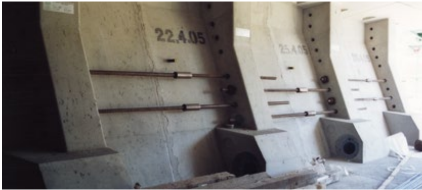
Typical Coupling, Uhlavu Bridge, Pilsen, Czech Republic
