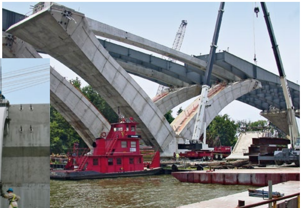
Woodrow Wilson Bridge, Washington, D.C., USA
